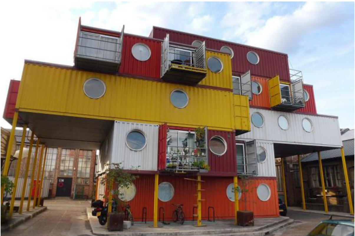
Container City 2 at Trinity Buoy Wharf, London in September 2012. Source: Urban Space Management (Container City) LTD
