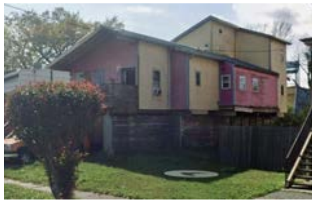
A dilapidated Make It Right Home. Source: Capital B
