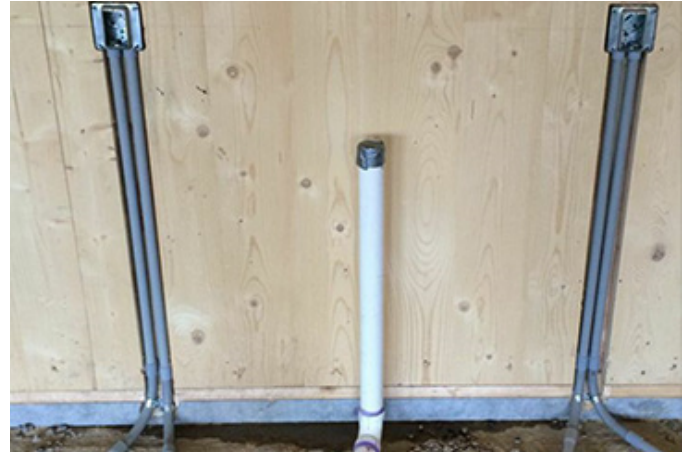
MEP cut flush into CLT wall. Source: Woodworks
