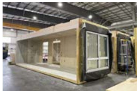
Module constructed with “punched out” wall. Source: Kalesnikoff
