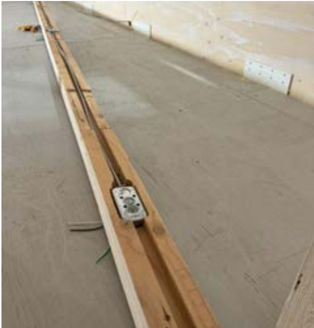
MEP strategy inside the home consisted of CNC-cut channels for electrical wiring, and enclosed cores hidden near the stairs. Door and window holes were cut into the thickness of the ply, eliminating headers.
