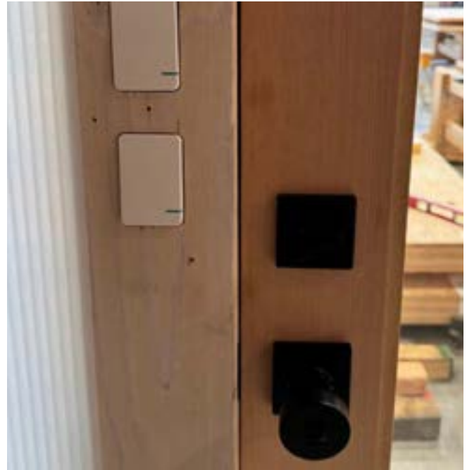
MEP strategy inside the home consisted of CNC-cut channels for electrical wiring, and enclosed cores hidden near the stairs. Door and window holes were cut into the thickness of the ply, eliminating headers.
