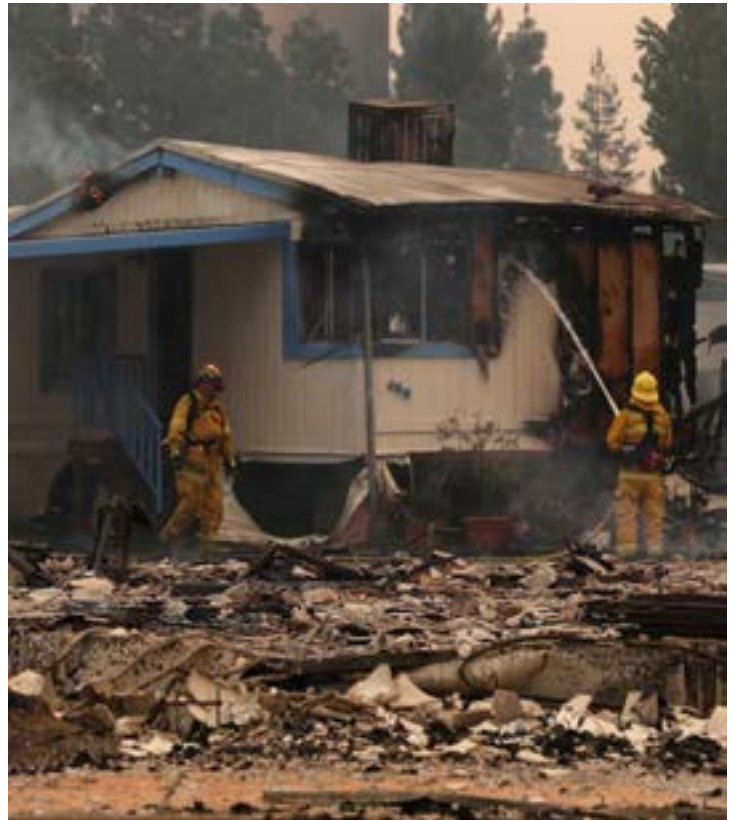
A fire damaged mobile home in Santa Rosa, California. Source: Justin Sullivan, Getty Images
