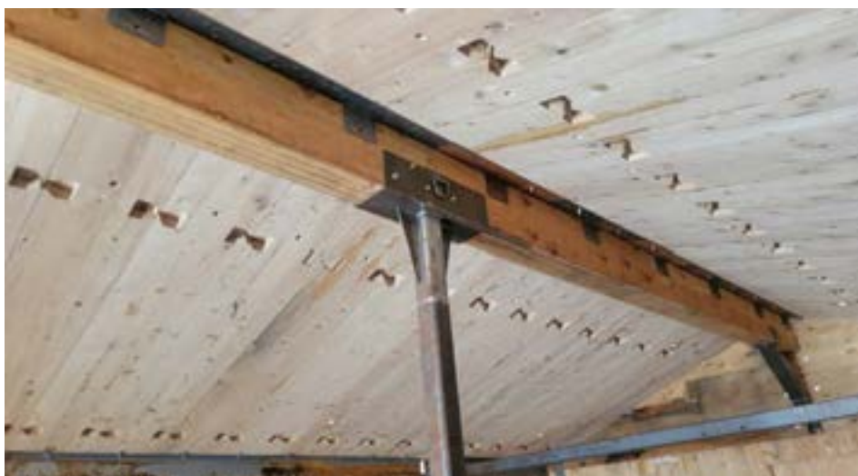
Exterior shots of the CLT B-Hut. Butterfly connectors provide shear resistance. The barrack model had recently been seismically tested.
