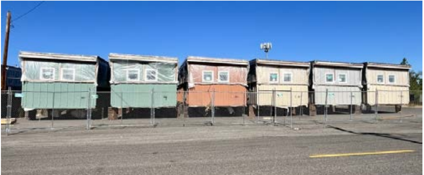
Decommissioned modular homes at Royal Oaks in Phoenix, Oregon. . Source: Jane Vaughan/JPR
