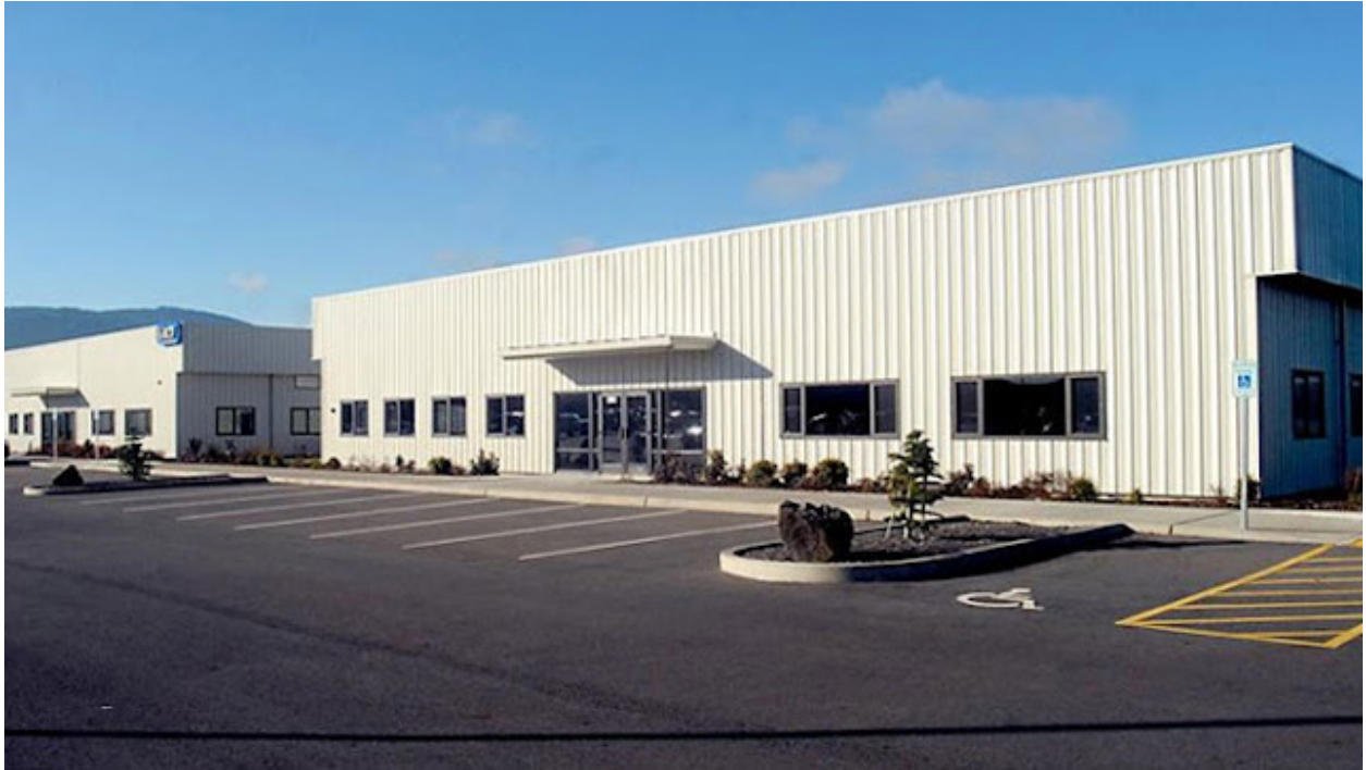
The Composite Recycling Technology Center. Source: CRTC
