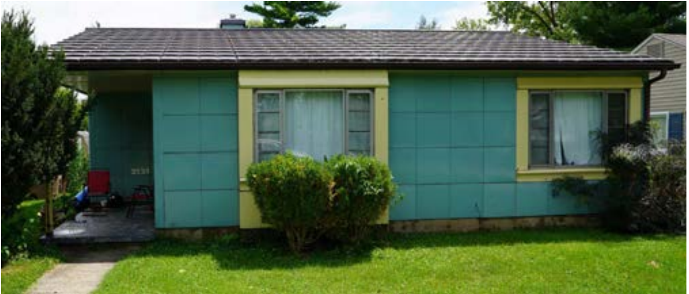
A typical Lustron House. Source: Quentin Melson
