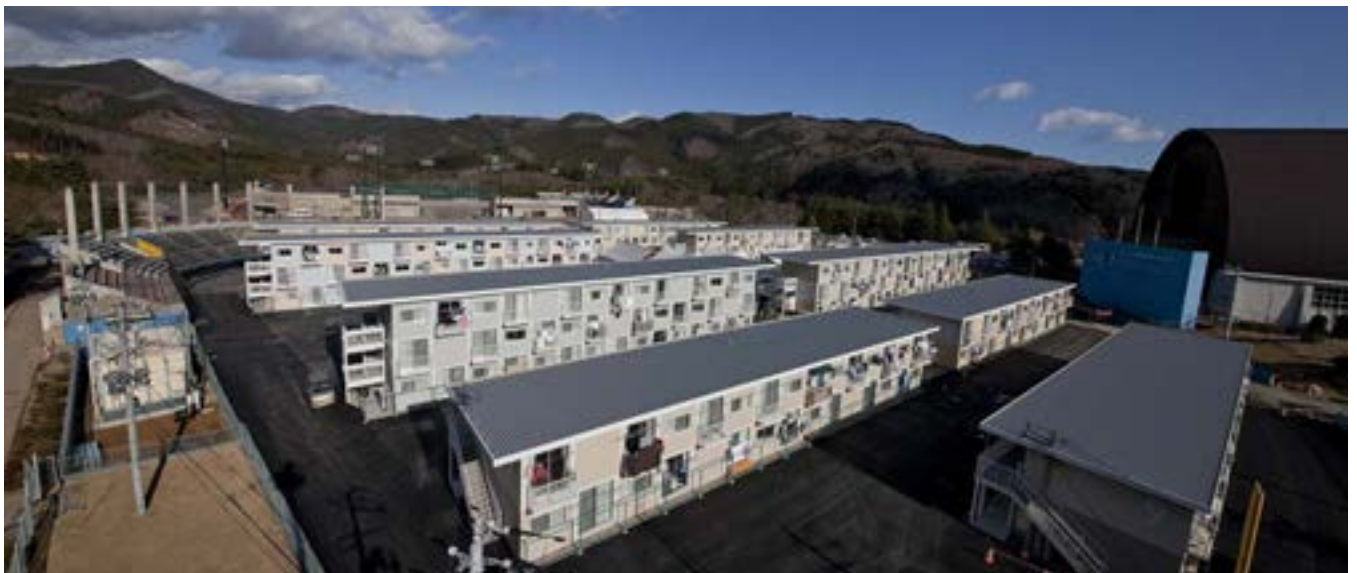
Three-story shipping container apartment buildings designed as temporary housing for Onagawa earthquake victims. Ban cited complaints about government issued temporary houses as an inspiration for the build. The homes include built in storage and finished interiors. Source: Shigeru Ban Architects
