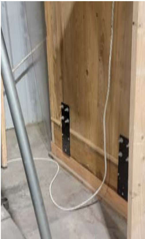
Interior and exterior wall-to-wall and wall-to-floor connectors, which use angle brackets, flat brackets, and tongue-in-groove cuts.
