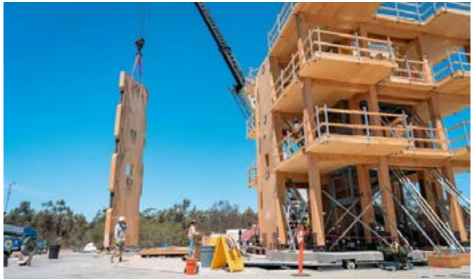
Seismic testing of 10-story structure by LEVER Architecture. Source: Building Design + Construction
