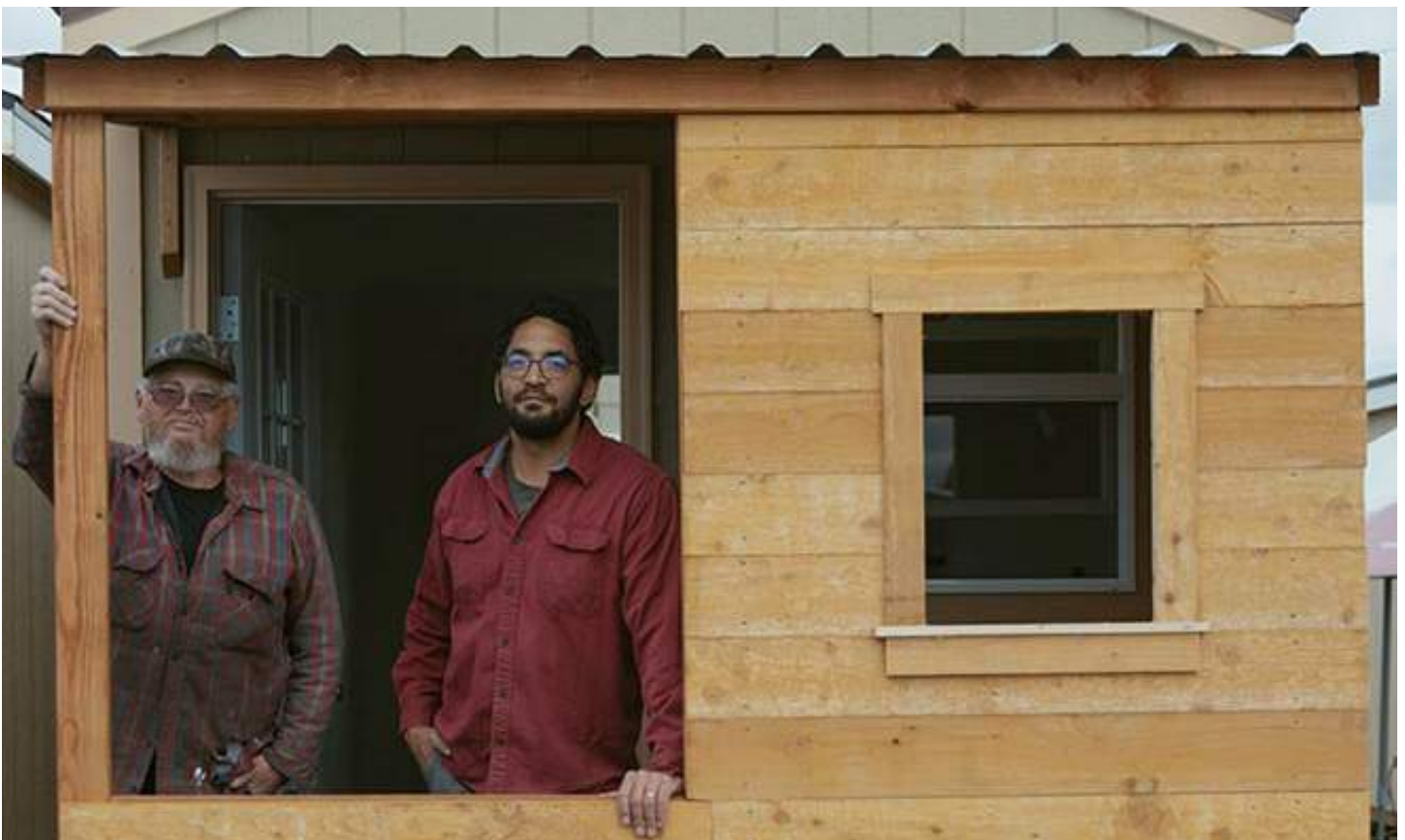
Villager Sam and Shop Lead Amiel frequently work together on projects like this cottage porch. Everyone Village, 2024.
