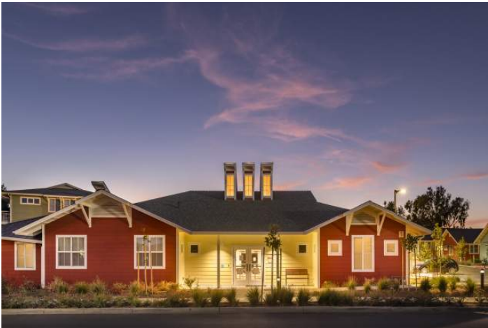
Valley View Community Club House. SAHA, 2022.
