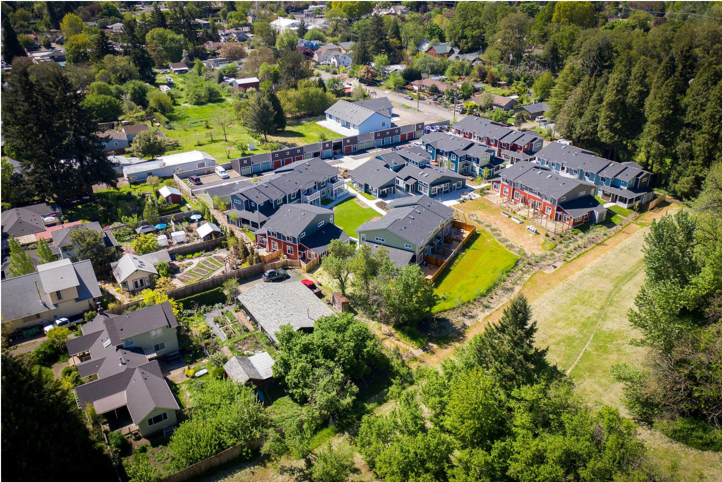
Aerial view looking west. Riversong Cohousing, 2022. Dixon, 2022.
